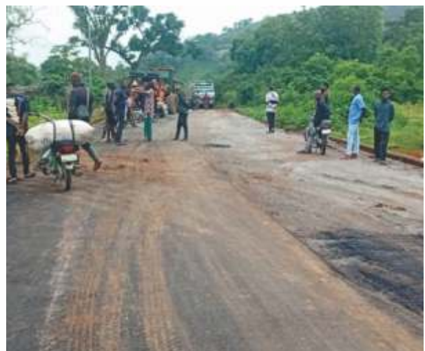
Asphalt laying of Oyi farm road
