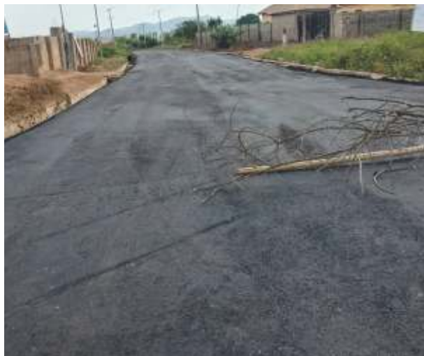
Asphalt laying of the road leading to the House of Olu Adde of Ekinrin-Adde
