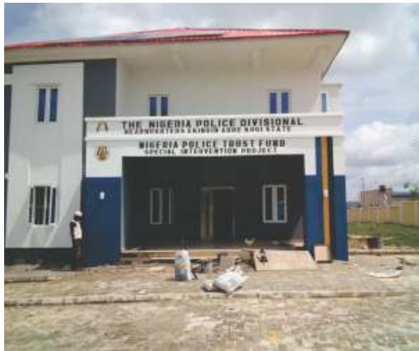
Modern Police Station
