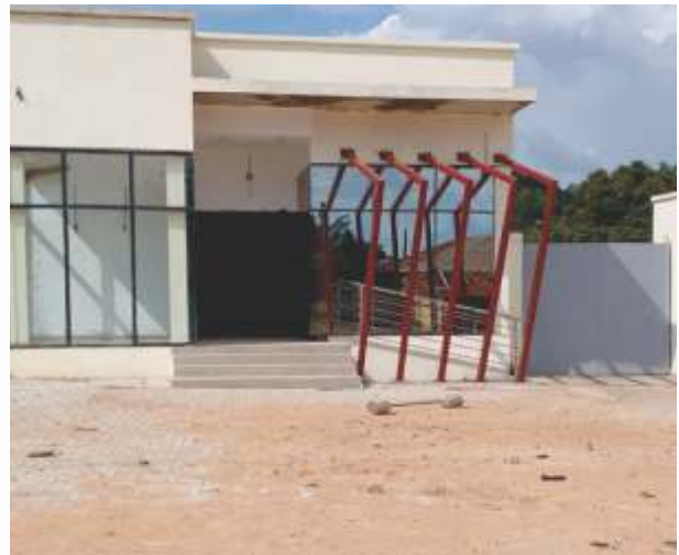
ACCESS Bank (under construction )
